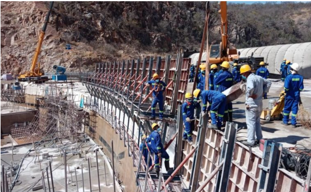
Construction of the Kunzwi Dam
