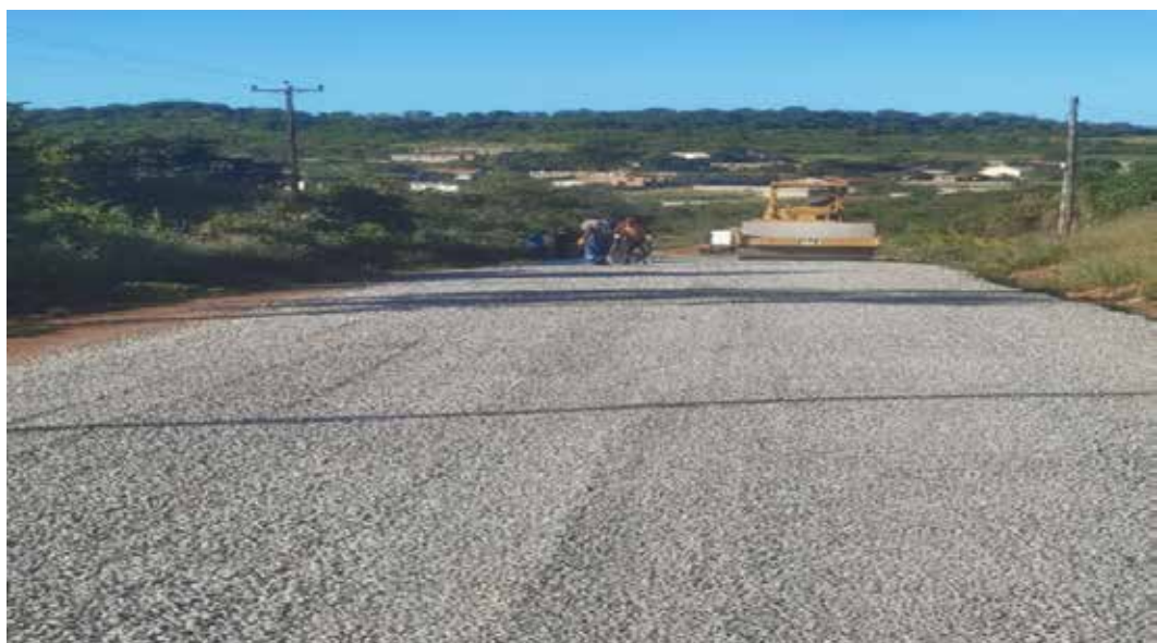
Gwanda Municipality, Jacaranda Road construction
