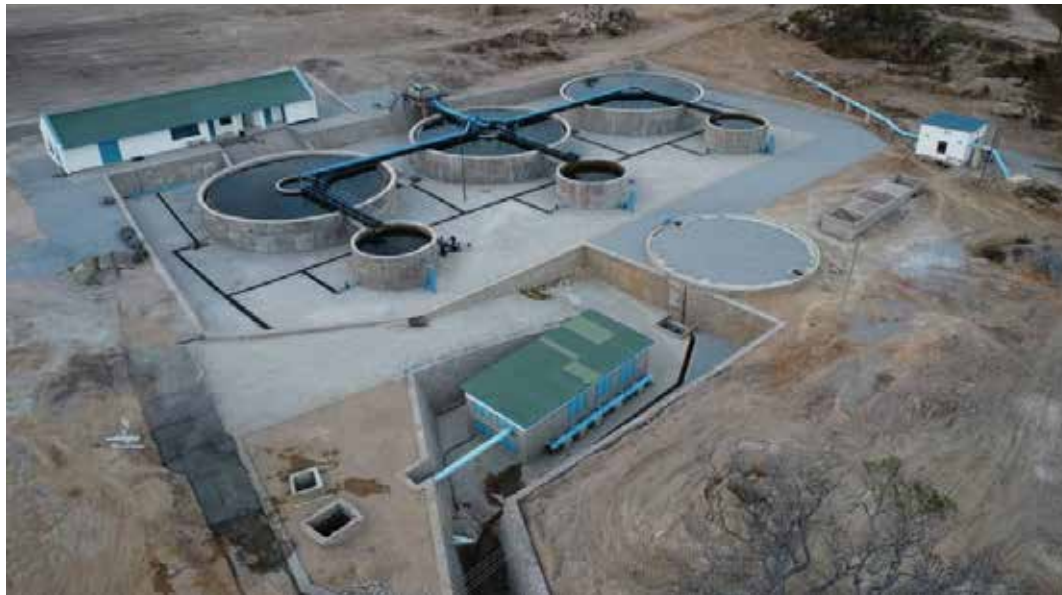
Chivu Dam Water Treatment Plant
