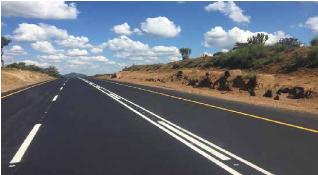
Completed section of the Harare-Masvingo-Beitbridge Highway
