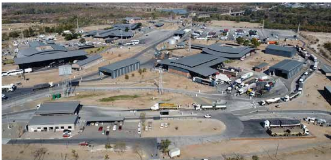
Renovated Beitbridge Border Post
