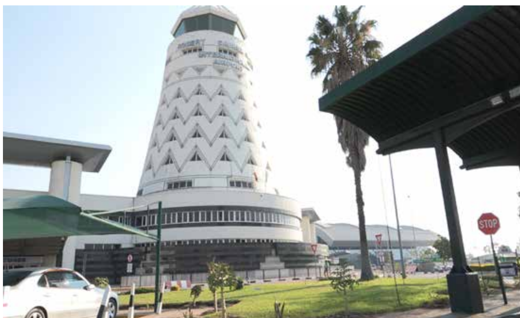
Renovated R.G. Mugabe International Airport
