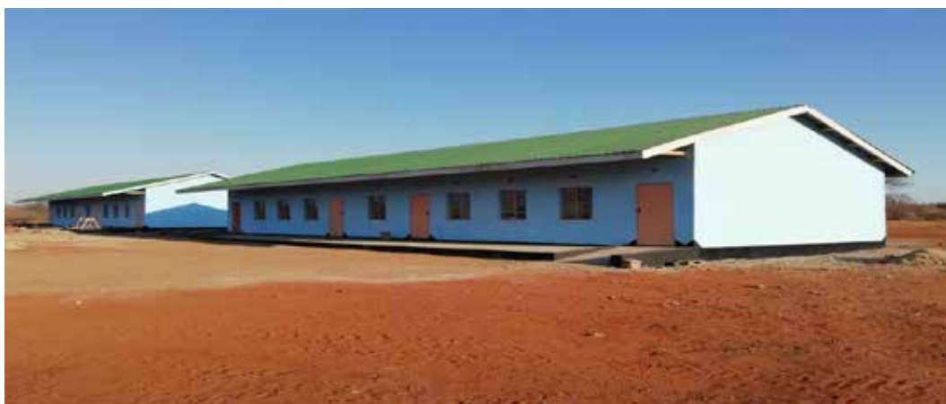
Novhe Primary School, Beitbridge RDC
